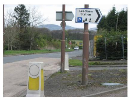
Traffic going straight over or turning right from the A6094 might have to be this close to the give-way lines to see well enough to the A703 to the left; suggesting the benefits which could arise from a review of the existing visibility splay. However, the original solution was expensive due to the lack of land available and the difficulty in obtaining the land required to improve the visibility splay.
