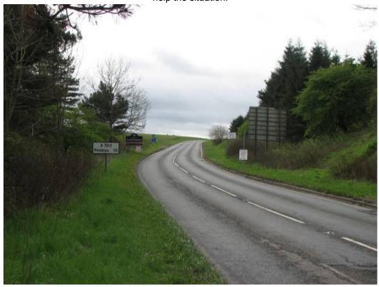
The A6094 approach is wide enough for 2 cars to sit side by side trying to enter the A703 and A701 and/or for traffic for the A703 to think they can go round bend fast – to reduce risk of A701 > A703 vehicles running into their back.
